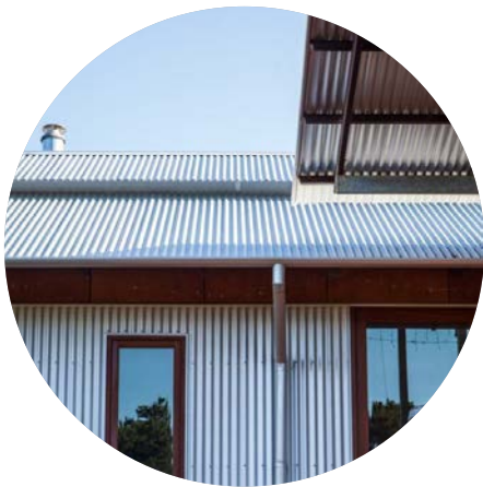
New cladding to Level 1 walls and roof
