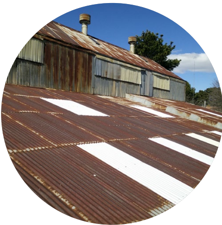
Reuse existing sheets for cladding
