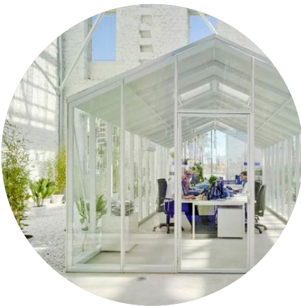
Fine steel and glass box added to shed
